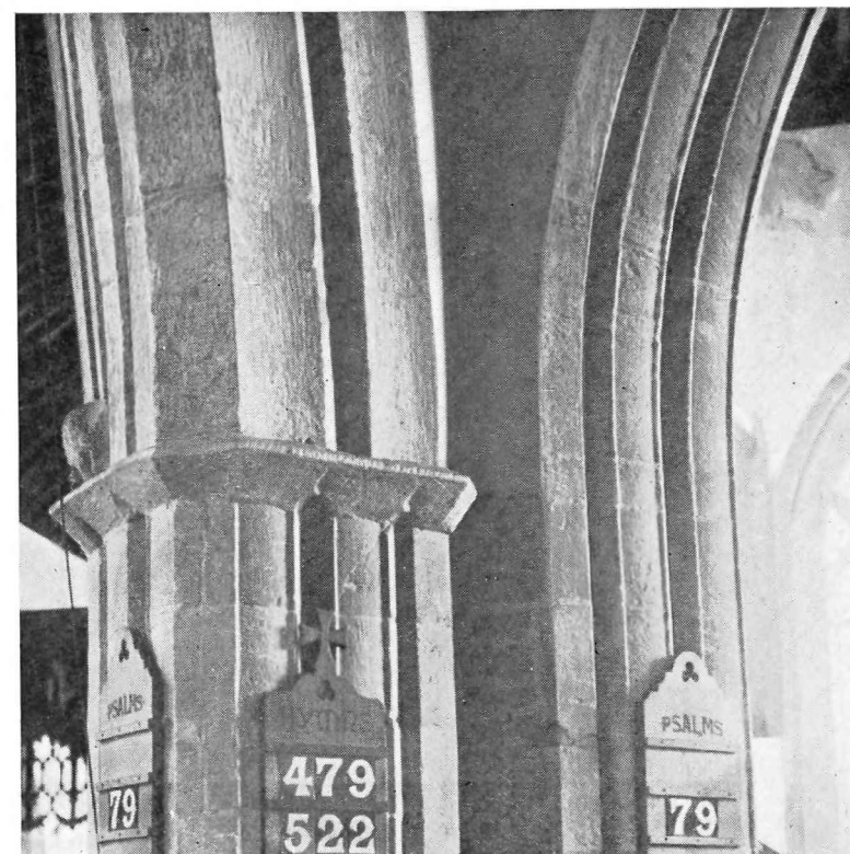
S.E. Pier of Nave (p. 42a).
