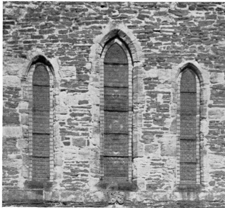
Windows above W. door (p. 43a). Late 12th-century.
