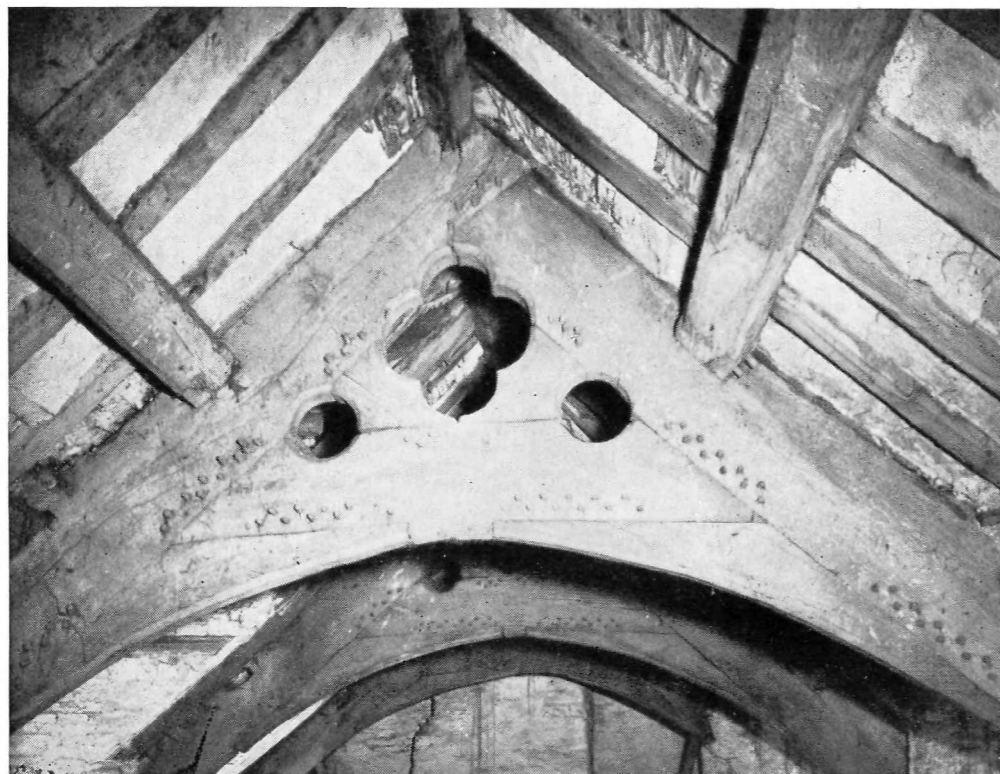
Plas-mawr (185, p. 62b), central block, hall roof. 1580.
