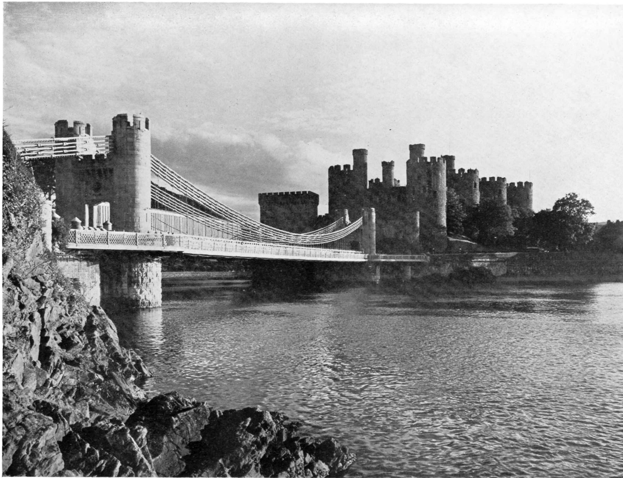
Conway Castle (183, p. 46b) and Suspension Bridge (198, p. 69b).
