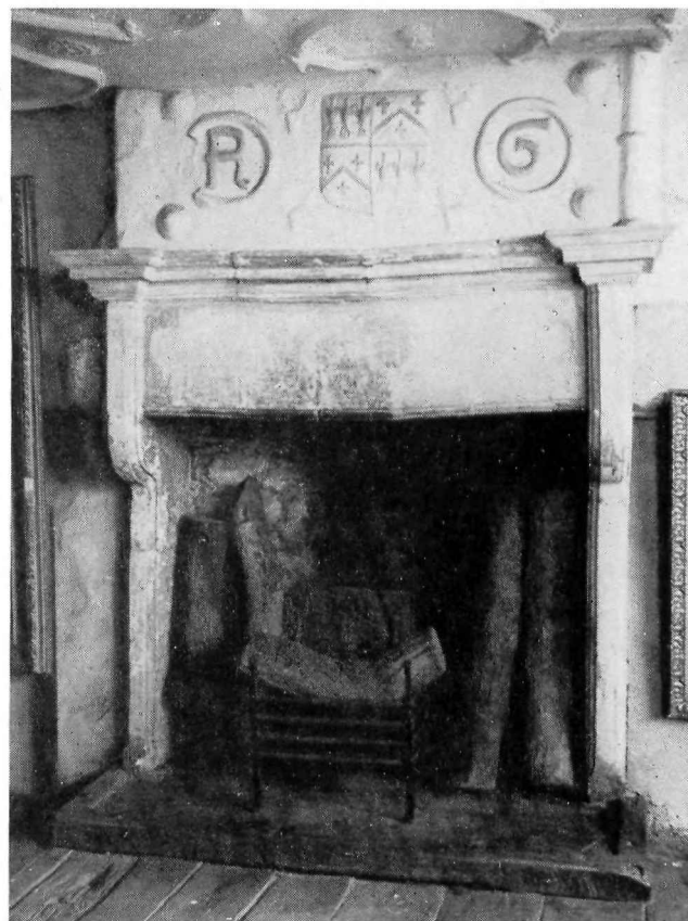
N.W. wing, first floor. 1576-7.
