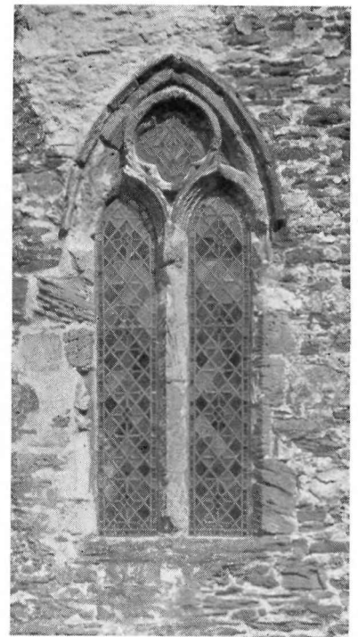
Window, S. wall of chancel (p. 41a). Ca. 1260.
