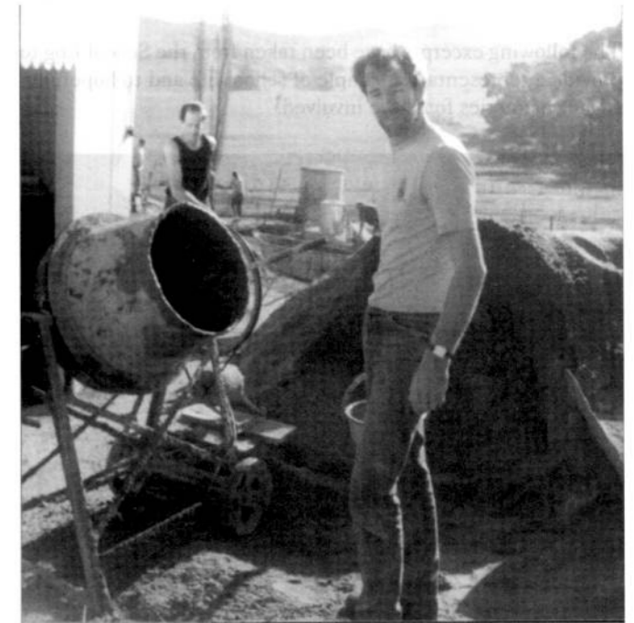
New swimming pool sheds being erected.
