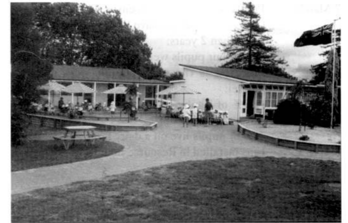
Cobbling and gardens by Room 4.
